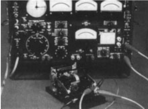
Testing of Protective Relays using a Relay Test Unit
